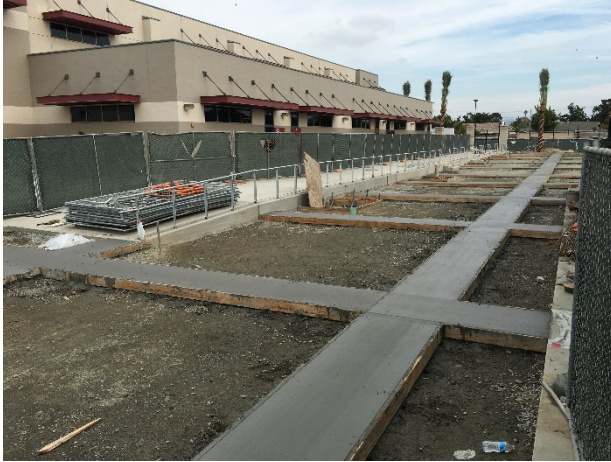
Installation of Phase C2 Walkway “Bands” Complete
