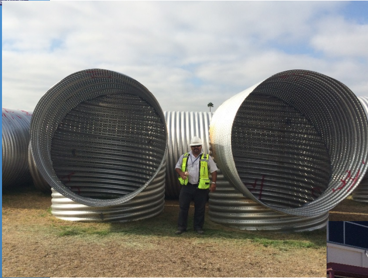
Detention Tank Piping
