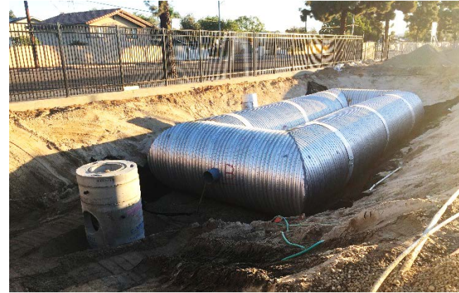
Installation of Infiltration System Piping – System D
