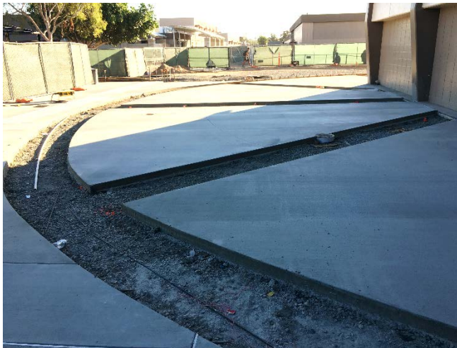
Radial Pattern Hardscape at Gym
