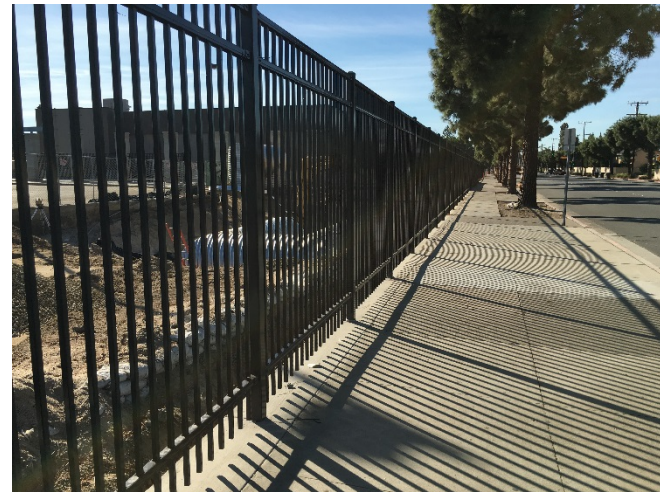
New Decorative Fence Along Wagner Avenue
