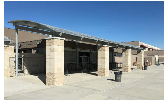
New Canopy and Hardscape at Food Service
