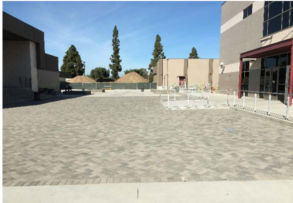
Phase C1 Pavers Complete
