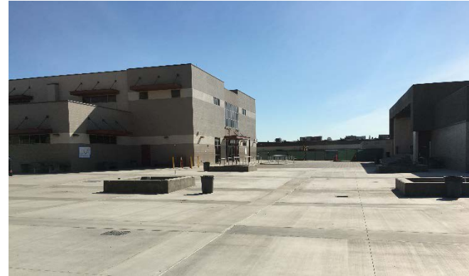
New Hardscape Looking South Towards Building E
