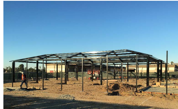
Shade Structure Framing Complete
