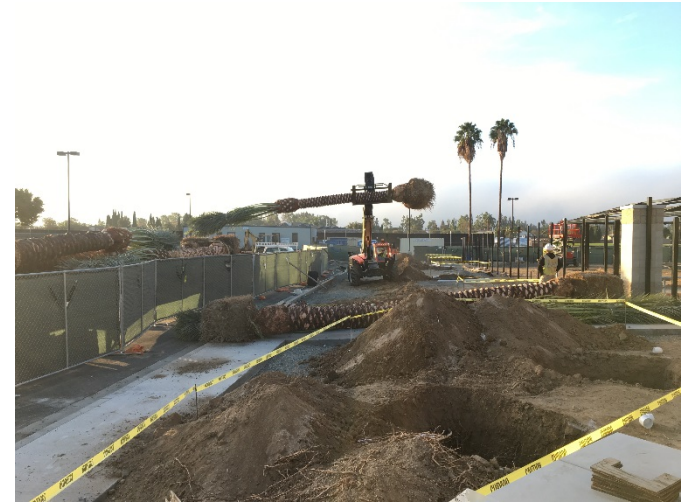
Installation of Palm Trees along Student Parking In Progress
