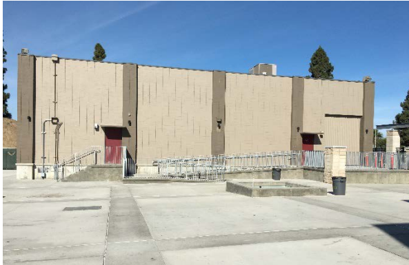
Hardscape and Planters Phase C1 North
